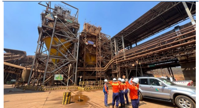
Exhibit 19. Nickel Matte Processing Plant
