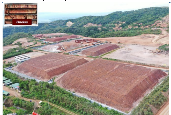
Exhibit 5. Heap leach plant under construction
