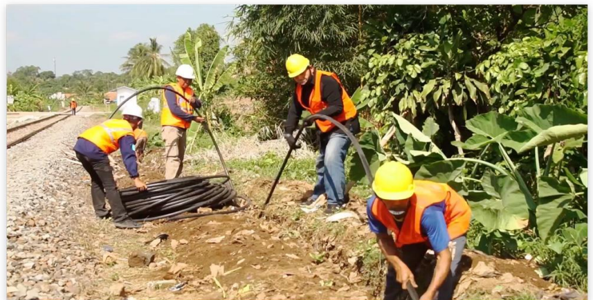
Exhibit 10b. Laying fiber cables alongside Kereta Api corridors
